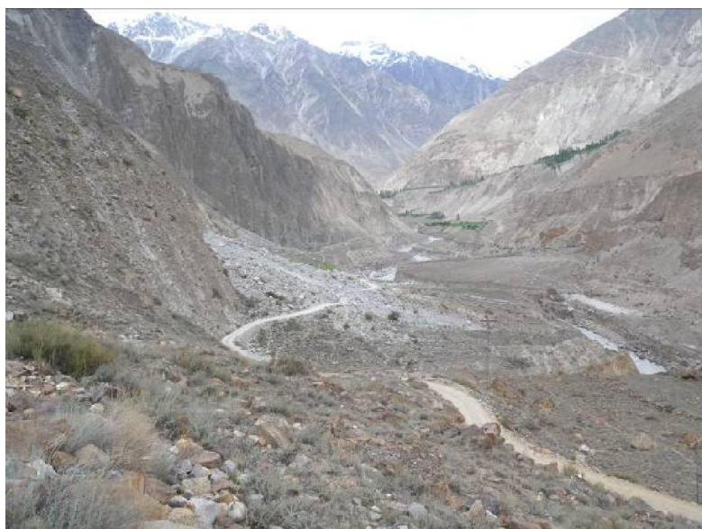
Exhibit 20 The debris flow recent deposits in light grey. During a landslide event, the debris completely flooded the road blocking its use.
