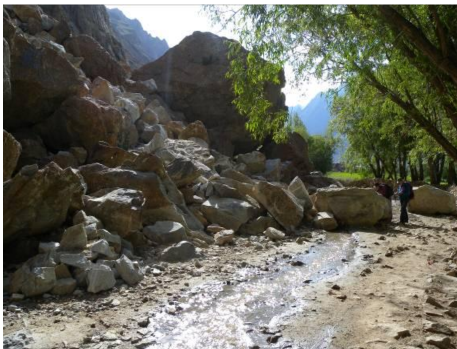
Exhibit 23 Rock fall at the beginning of the track to Concordia (K2 Base Camp). Boulders partially occupied the track. The first part of the track leading to the Biafo Glacier is subjected to rock fall phenomena. Some of them occurred also while the researchers were surveying. Boulders are present in the area and in the 90% of the cases their runout distances are intercepting and crossing the track.
