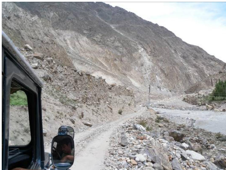
Exhibit 19 Rotational landslide in fluvio-glacial deposit. The event caused damage to the infrastructure present in the area making it unstable for a period. Fluvial banks are subjected to high toe erosion that is the main cause of landslides. There are no mitigation measures to avoid erosion along the fluvial banks.
