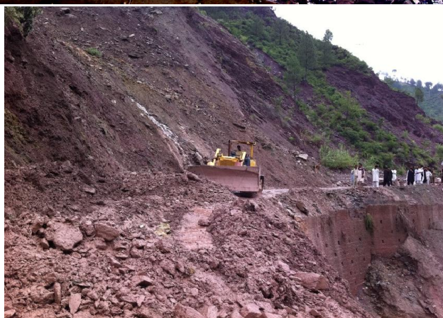
Annex 4-10: A) Landslide along the Neelum River due to Seismic Activity of 2005 (Debris Fall); B) Debris Flows.
