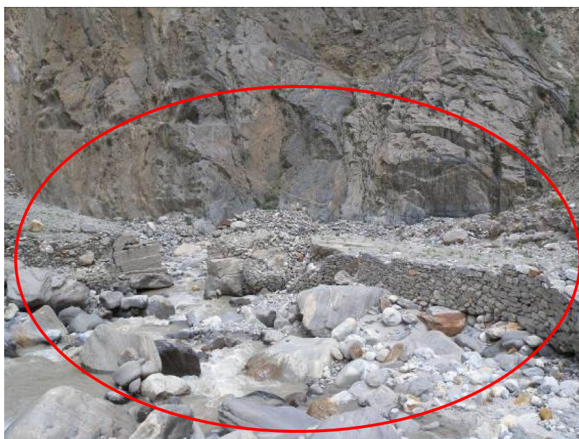
Exhibit 21 From upstream to downstream, an example of the damages caused by a debris flow to the road. The road crossing has been completely flooded away.
