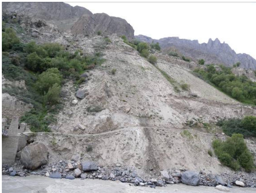
Exhibit 22 Rotational landslide in colluviums. The morphology helps in indicating the landslide dimension and highlights the safety of the built road.
